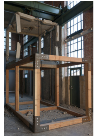
The Power Station Dallas, United States
